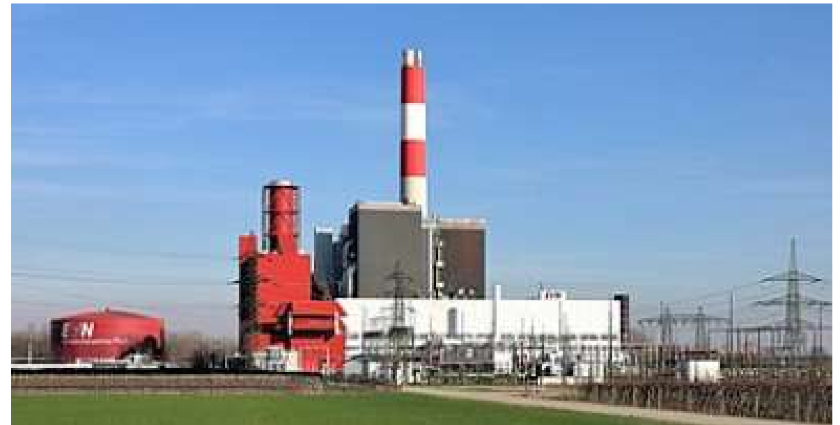
Theiss power station – EVN AG (Wärmekraftwerk Theiß (800 MW))
